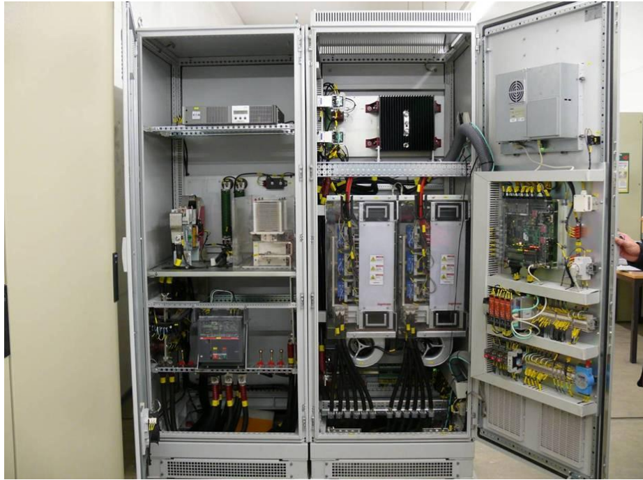
Figure 27: View and technical principle of the INGETEAM inverter in substation Oetkerhalle
